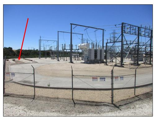
**Photo 1:** View looking southeast at the existing Templeton Substation. Note the concrete-lined detention basin in the southern portion of the substation (red arrow).
